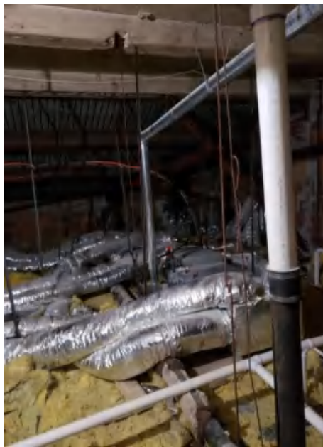
Furnace in Attic Space
