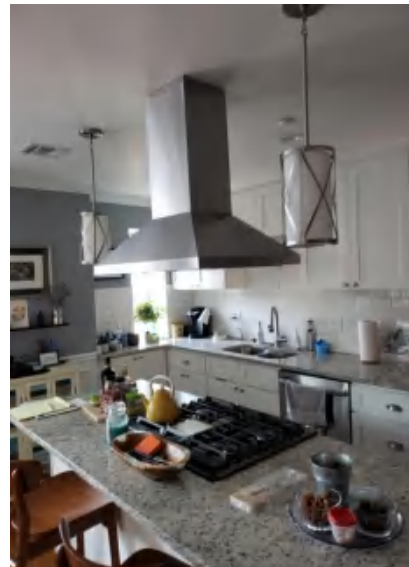
Typical Kitchen Hood
