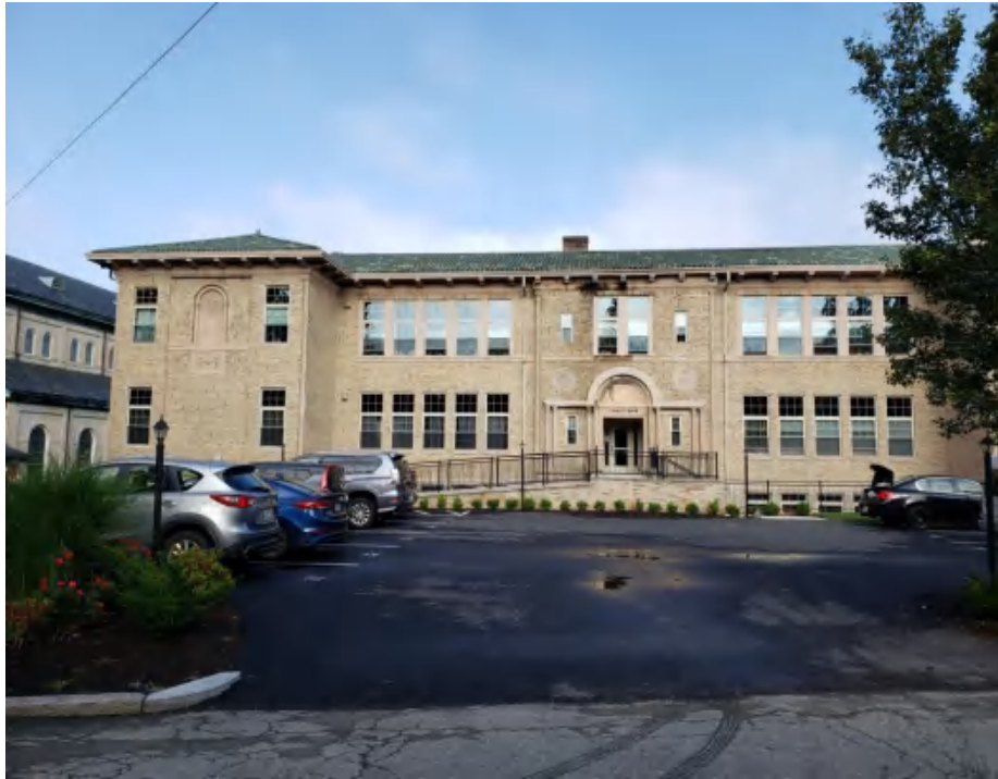
Front of Building
